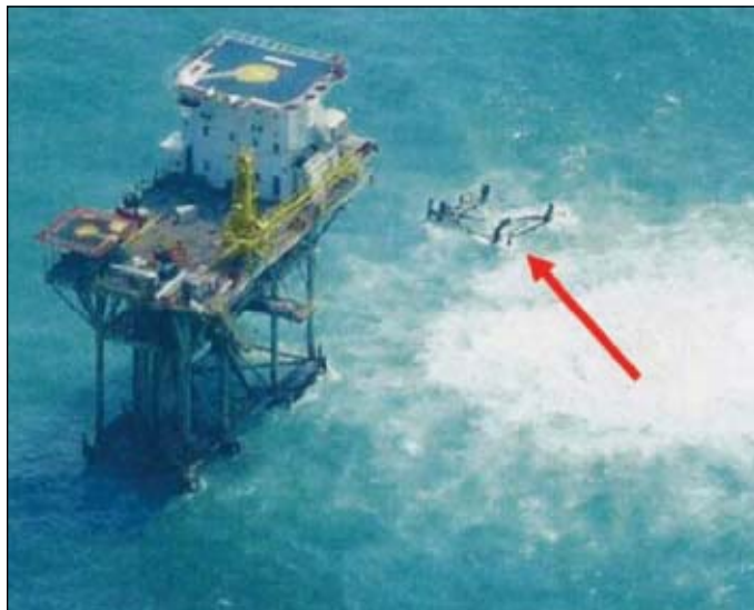
A hurricane destroyed this platform in the East Cameron Area (Fig. 2). Photo from US Minerals Management Service.
